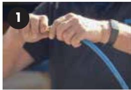
**1** Determine where the hose is damaged
