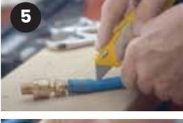
**5** Cut the hose at the end where the remaining part of the FastFix fitting is
